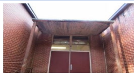
Corroded Steel Canopy
