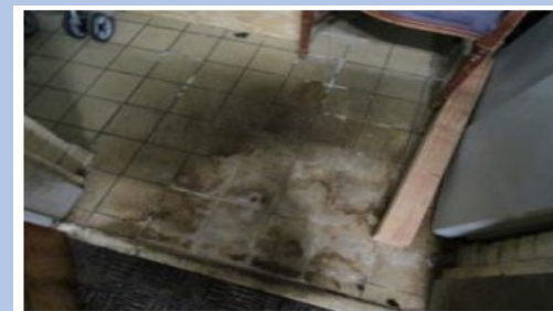
Damaged Quarry Tile Flooring
