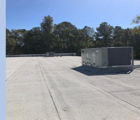
After Unit Placement
