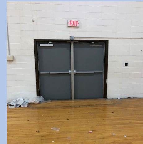
New doors in gym
