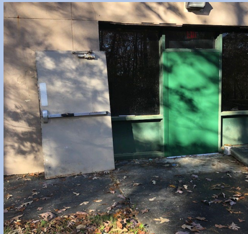
New door (green) with existing door new
