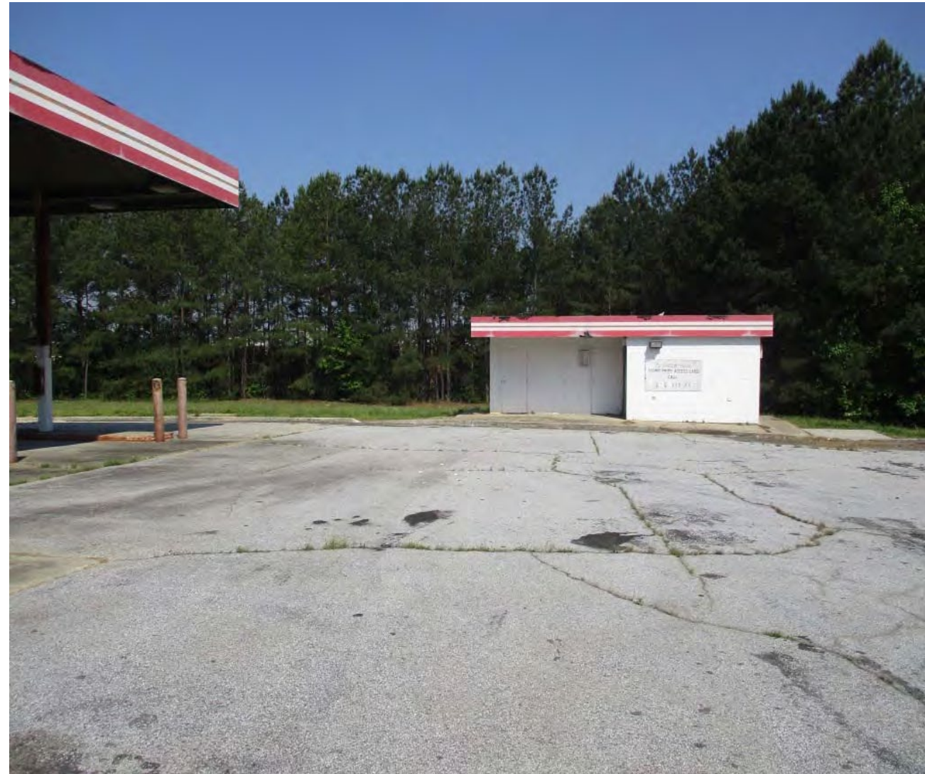
Canopy, pavement and vacant building facing NW
