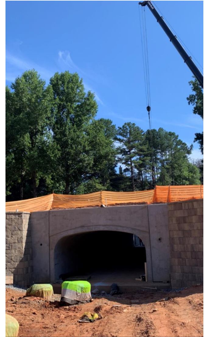
EXAMPLE OF TUNNEL UNDER MERK AND BUTNER ROADS (BIG CREEK GREENWAY)
