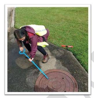
Each segment of the stormwater system is regularly inspected. Here, a top is being removed to check for obstructions and leaks. This is Highland Hill Drive.
