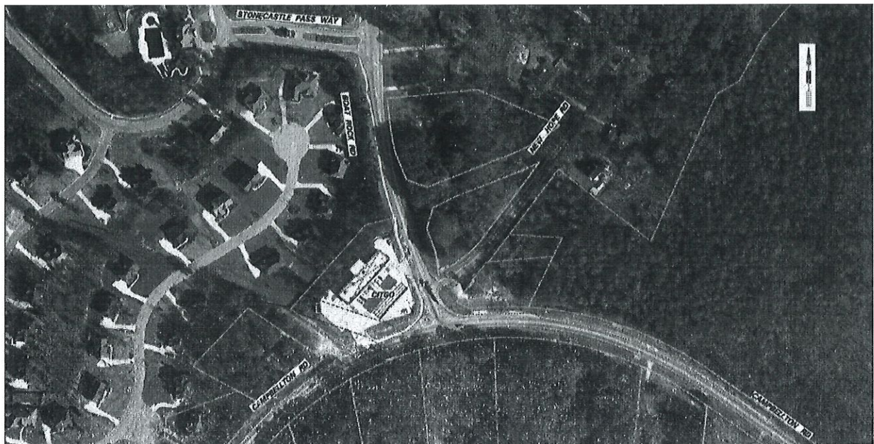
Figure 1. Existing Campbellton Road (SR154/166)/Boat Rock Road and Boat Rock Road /New Hope Road Intersections
